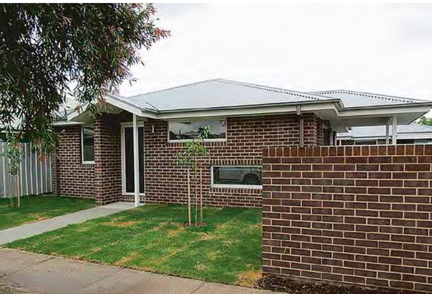
Recently completed one bedroom property funded by the Victorian Property Fund.
